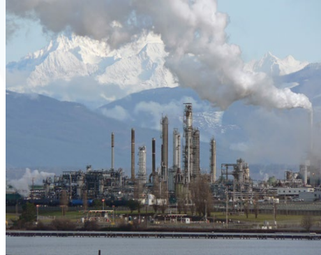
Refinery Off Gas
