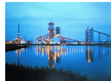
Next Generation Power Plants
