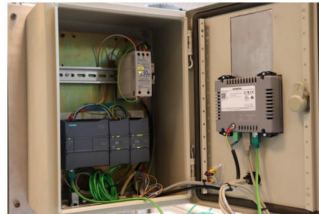
(c) Low level control system based on the Siemens S7-1200 platform.
