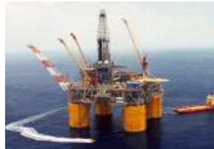
Fig. 4: A typical TLP facility 2
